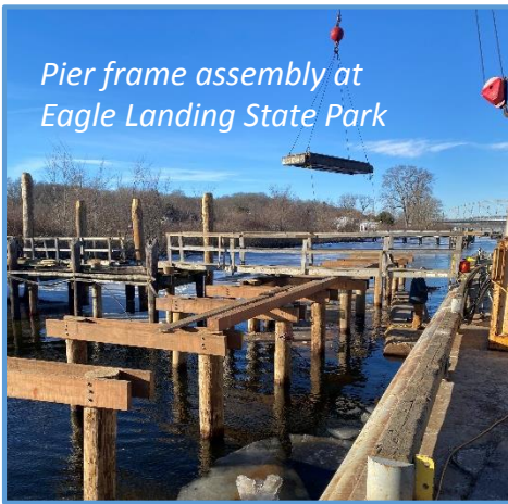
Pier frame assembly at Eagle Landing State Park
