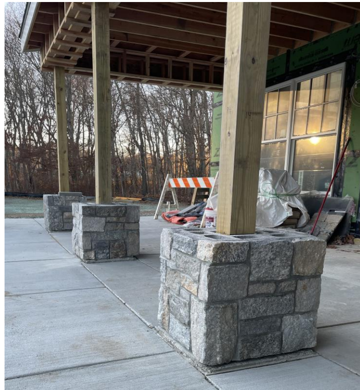
Masonry at Covered Porch Columns
