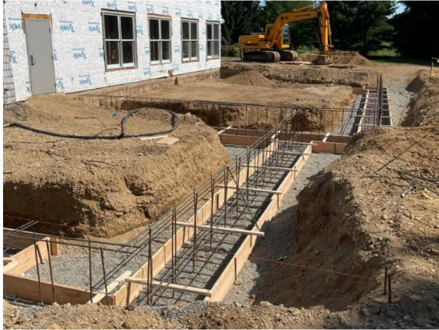
Concrete forms and rebar for the West addition footings
