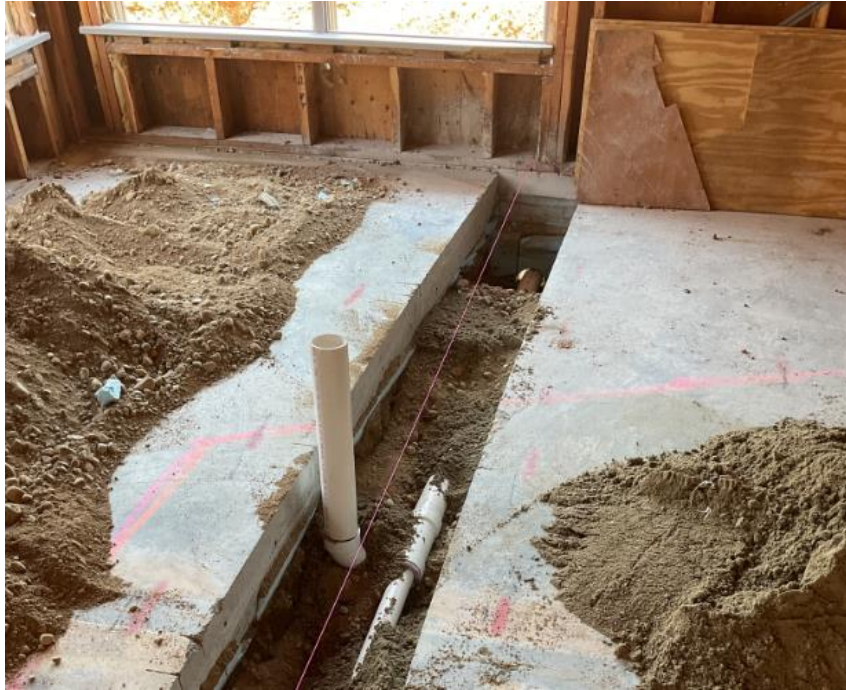
Underground plumbing for new Craft & Multi Purpose room
