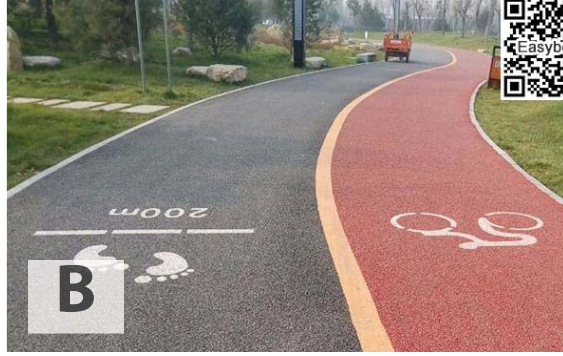
B Asphalt with Color Seal
