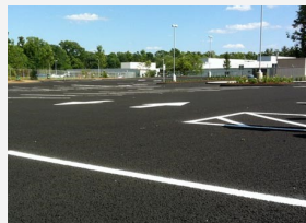
Pervious asphalt at Goodwin College
