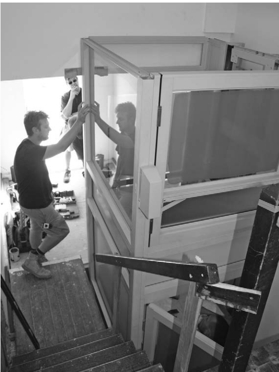
Handicap platform lift installation at the Old Lyme Historical Society
