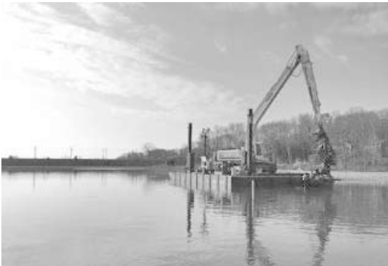
Below: Three pictures of the in-river dredge rig
